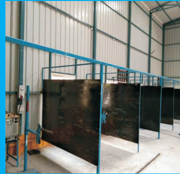
WELDING BOOTHS VIEW
